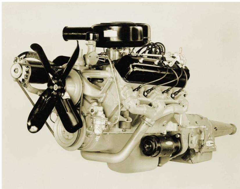
Eighteen bolts secure each cylinder head, more than most competitors. Head gasket issues were and have been virtually nonexistent, even when the engine was first supercharged for some 1957 models.
